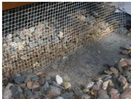
Animals can be excluded from under decks and sheds by placing small mesh fencing along the bottom edge and outward as shown. Landscape rocks or turf should be placed on top of the fencing that is flat on the ground
